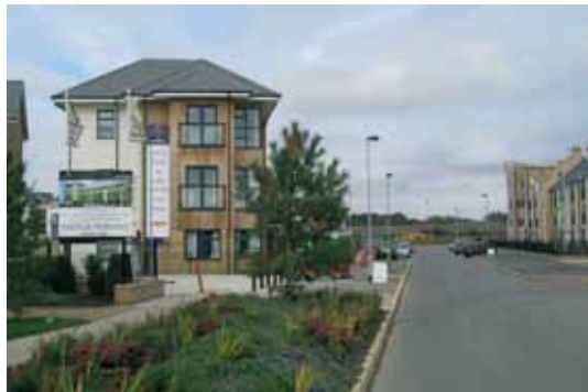
Orchard Park is incomplete. A14 in distance
